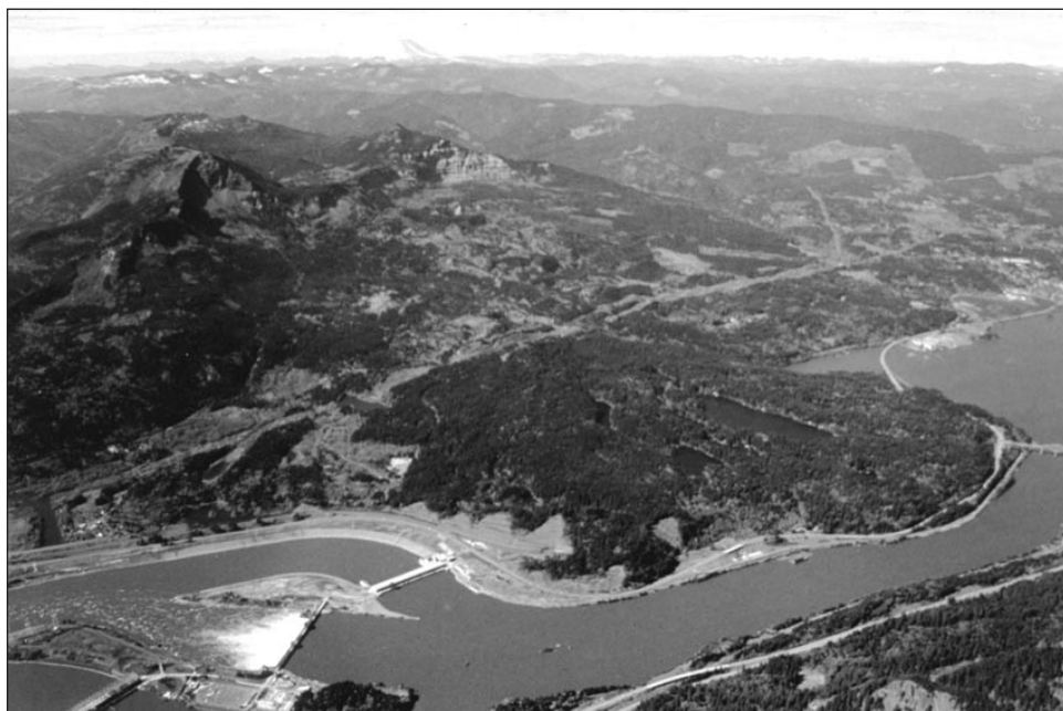
Figure 1. Aerial-oblique photo of the Bonneville landslide. View is to the northeast with Mount Adams volcano in the distance. Table Mountain with its triangular scarp is in the upper left of the photo. Bonneville Dam and its powerhouses (lower left) and the ‘Bridge of the Gods’ highway bridge (far right) flank the landslide. Photo courtesy of Derek Cornforth, Landslide Technology .
