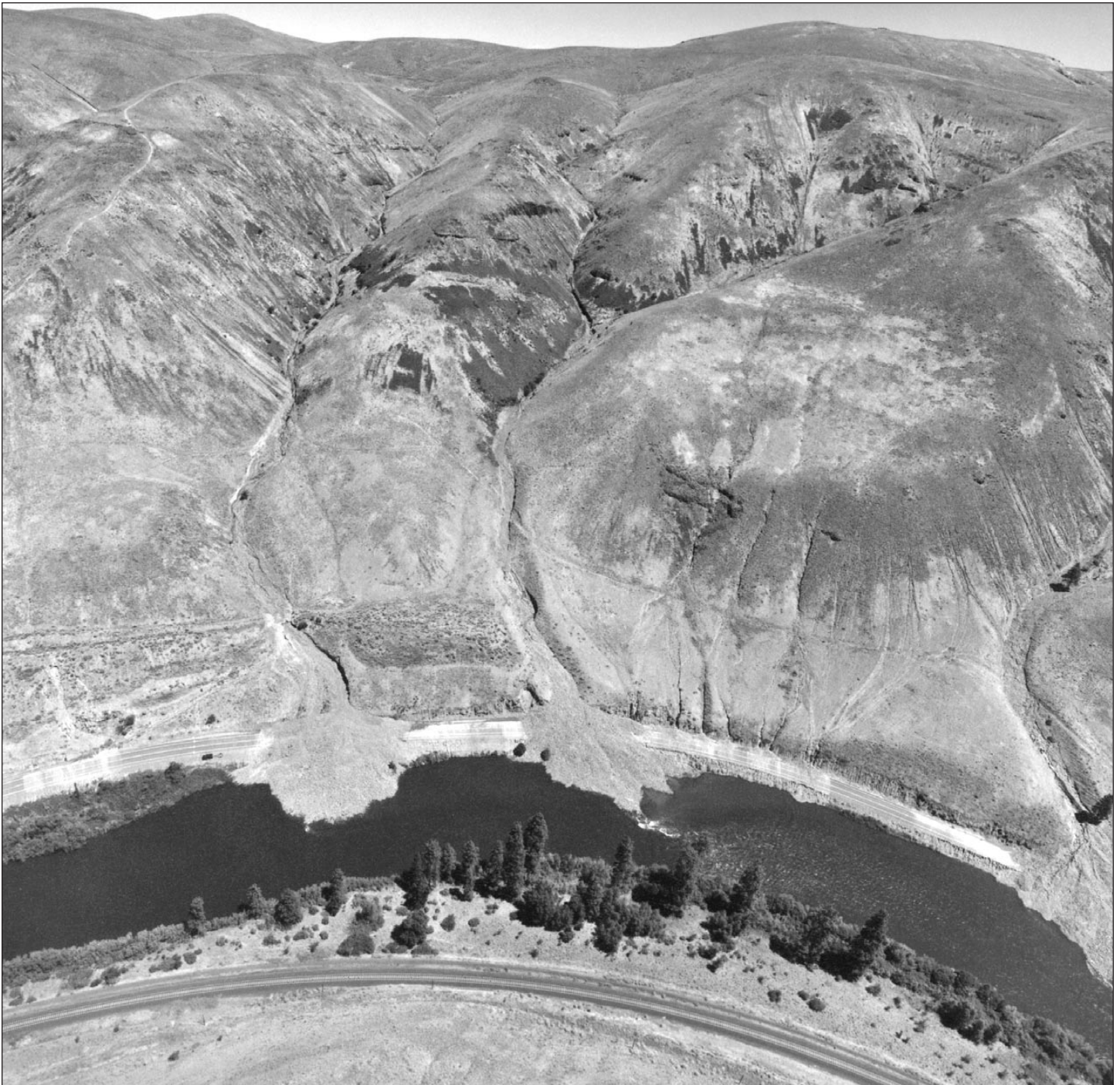
Figure 3. Debris flows along the north side of Beavertail Bend of the Yakima River burying State Route 821 and debouching into the river. Note the small catchment areas of the ravines and their steep scoured channels. Photo courtesy of the Washington State Department of Transportation.
