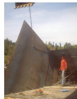
Welders finish the cap to the shaft.
