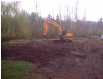
A track-hoe demolished the house and dug out the septic tank.
